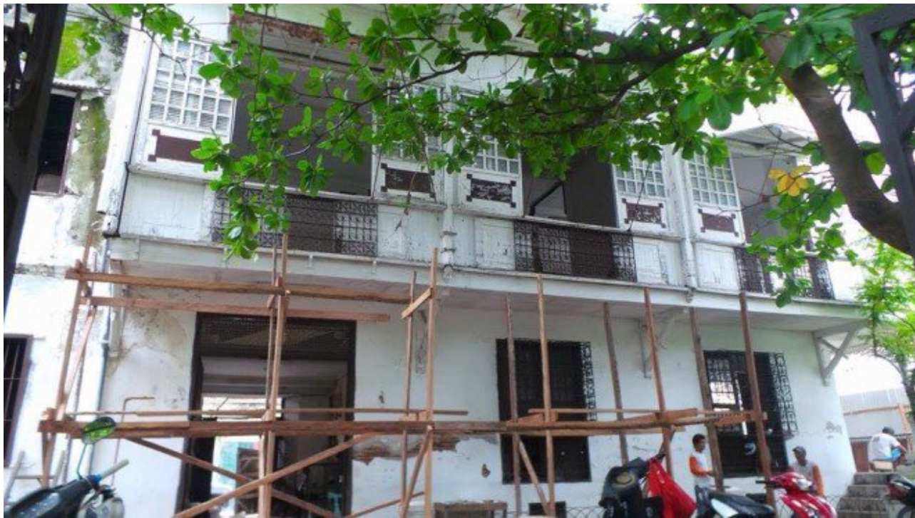
Before demolition —PHOTOS COURTESY RAYMOND DE VERA
