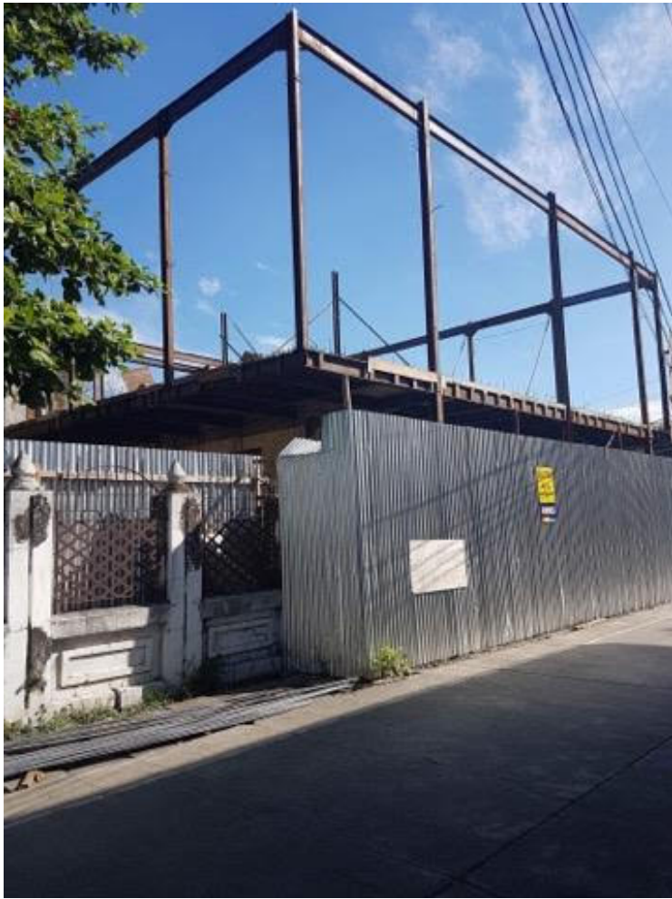
What's left after demolition
